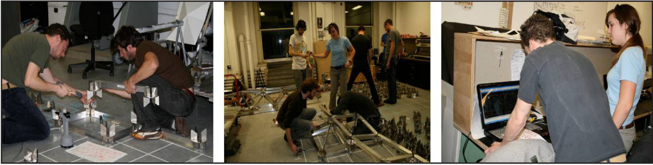
Fig. 6: Assembly of units at GSAPP
